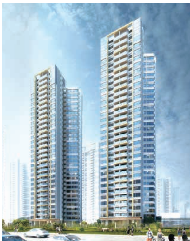
Jinghai Site No. 02, Jianghai District, Jiangmen
